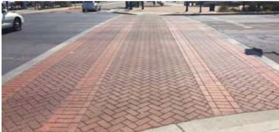
Existing LRT Downtown Crosswalk Pattern
